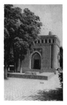
until now. The monument's composition is very simple and laconic. It is presented by a cube covered with a semi-circular larger dome and four smaller domes. Its rectangular is oriented to the cardinal points. The building is placed on the low socle and is completed with the arched gallery surrounding its top.
