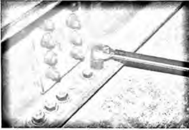
Fig. 7. Bolt tightening by a torque wrench
