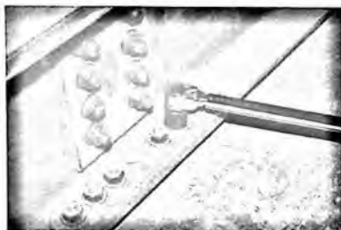
Fig. 7. Bolt tightening by a torque wrench
