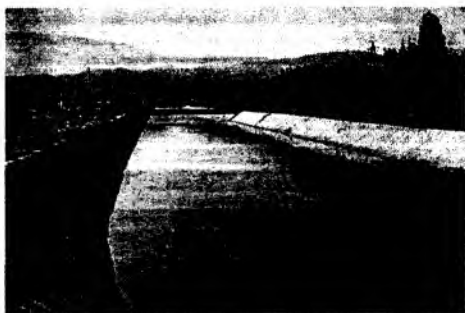
59-rasm. Yaxlit beton to'shamali kanal.
